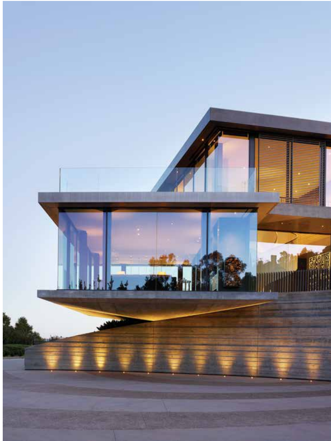
After visiting Frank Lloyd Wright’s Falling Water, Kirkpatrick conceived the sinuous board-formed concrete base below Balance Hill’s cantilevered, rectilinear living room, which soars dramatically above the Los Angeles basin. Photo: Richard Powers
